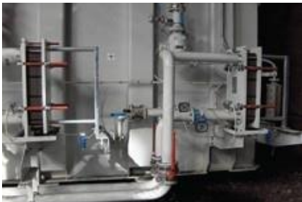
Plate and tube heat exchanger
