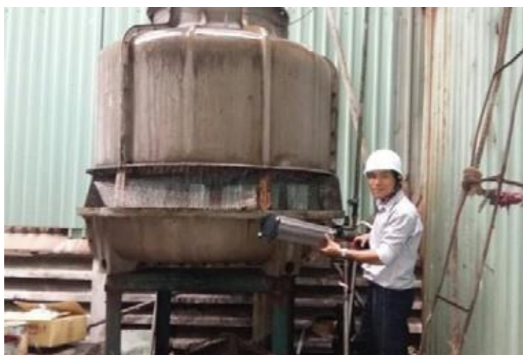
Prepare equipment into the cooling tower
