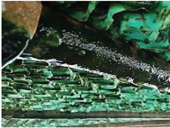
Algae reduces heat exchange efficiency
